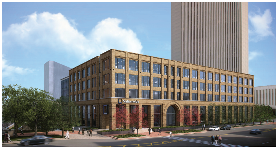
The planned Nationwide office building, set to bring 1,000 workers downtown to the Arena District.
